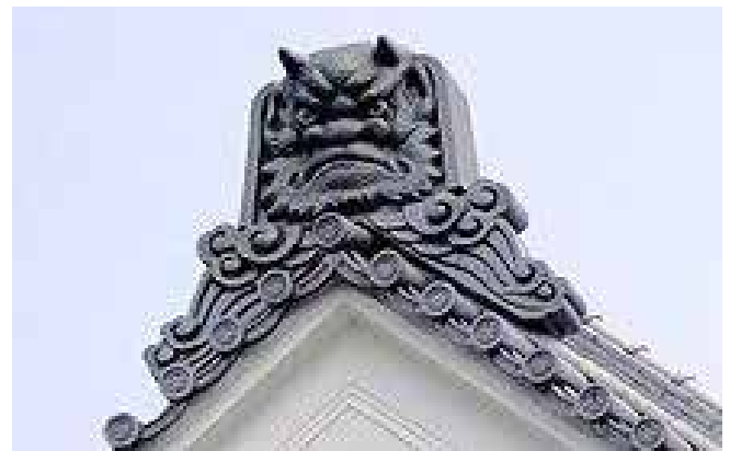
Onigawara on the roof of Tokyo National University of Fine Arts and Music.
